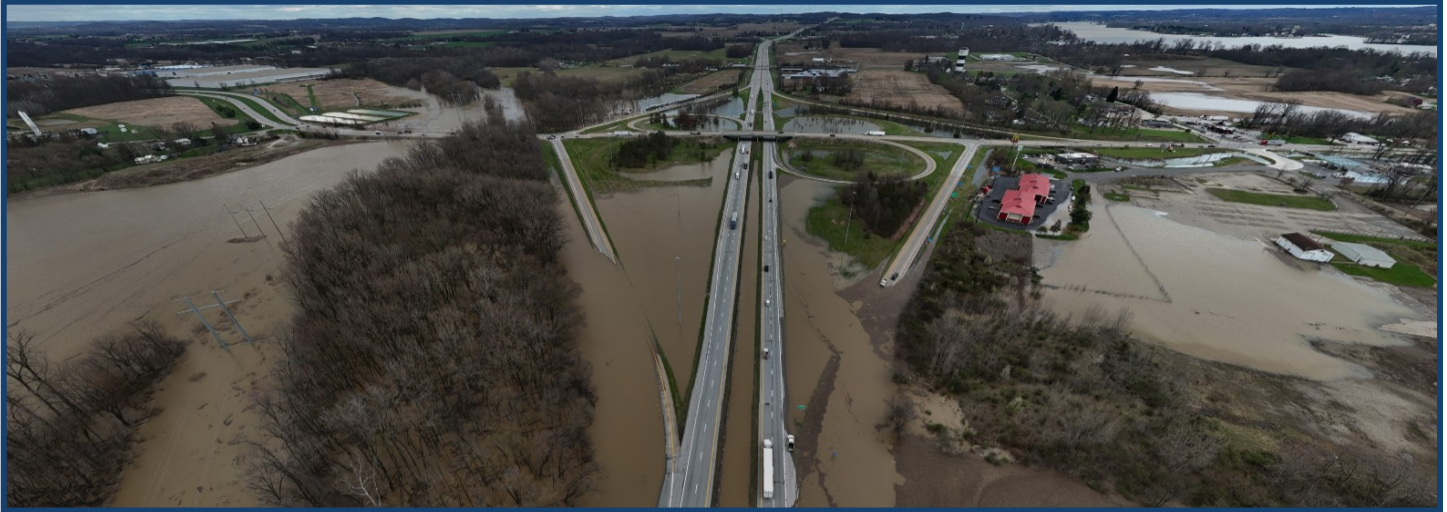
Figure x: I-70 Flooding. Photo Source: Gannett Fleming Engineers & Architects Drone photography
